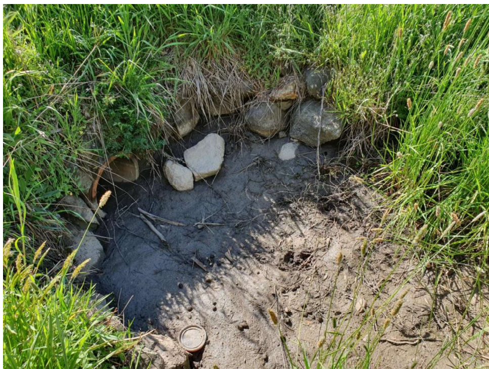
Photograph 4: stormwater drain located in the central portion of the site. The drainage channels are anticipated to be a collection point for lead and PAH contamination with sediment runoff during heavy rainfall events.
